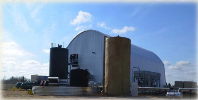
Sister Company Pilot Plant, Alberta, Canada
