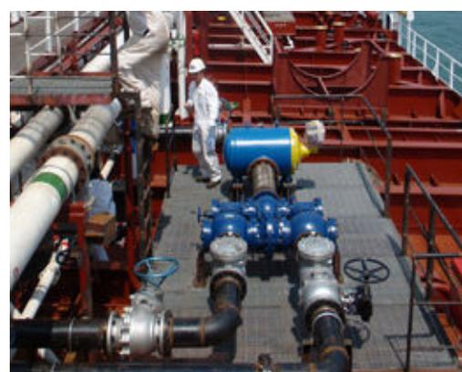
Figure 4 - barge mounted blender with PD flow meters – Source CBI
