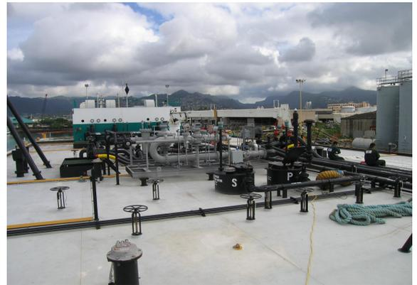
Figure 3 - Barge mounted in-line blender – Source Jiskoot
